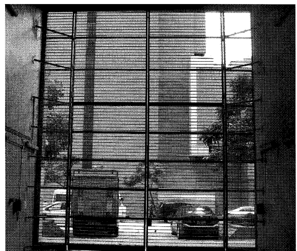
Figure 15 Improvement of Transformer Bay Ventilation by Door Gate Replacement
