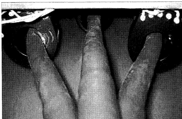
Figure 4 PD Detected on Cable Termination by Portable PD Detector
