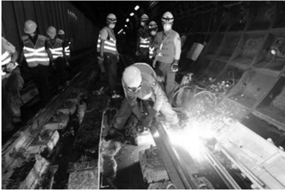
Figure 11 Installing New Turnout
