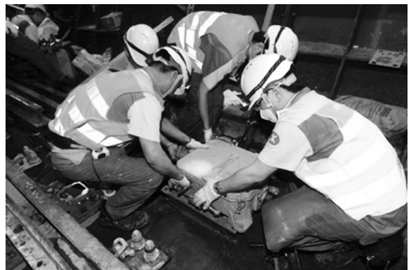
Figure 14 Installing New Trackside Signalling Equipment
