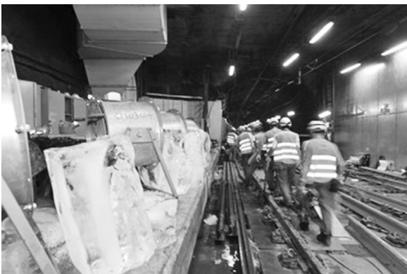
Figure 15 Cooling System for Work Site
