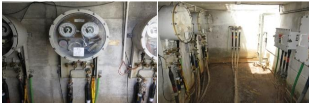
Fig. 4 - Gauge panel in underground pit
