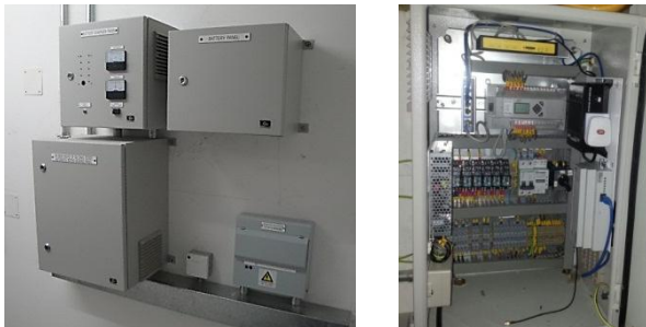
Fig.16 - AMR Outstation in residential building
