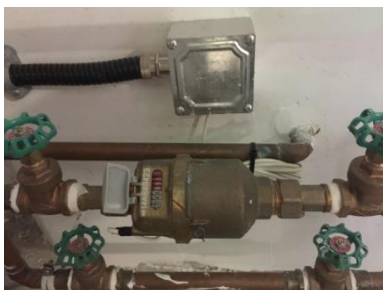
Fig.3 - Trial use of mechanical water meter with reed switch in WSD
