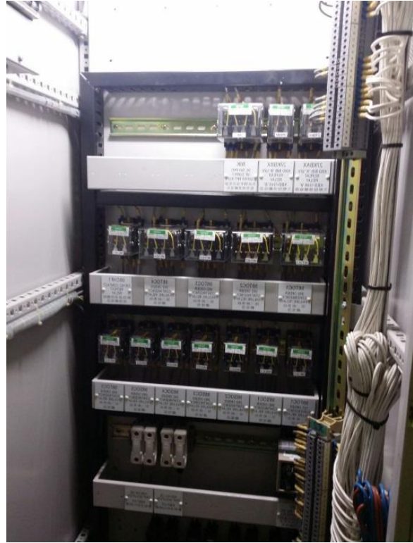
Fig. 1.2 – General appearance of 33kV automatic changeover and interlocking relay panel
