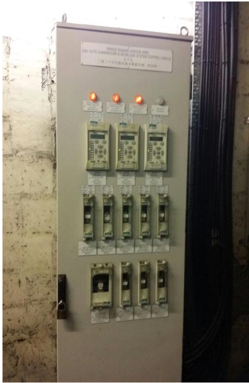
Fig. 1.2 – General appearance of 33kV automatic changeover and interlocking relay panel
