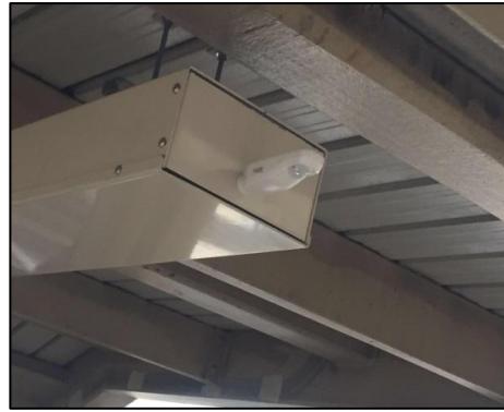
Fig. 10 - Motion sensor installed at Footbridge KF77, Choi Hung
