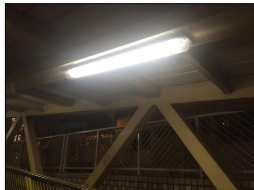
Fig. 7 - T5 LED tube lighting fitting at Footbridge KF77, Choi Hung
