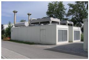
Fig. 24 - Outdoor D-UPS Installation
