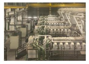
Fig. 1 - 11kV Diesel Generators in Generator House 1 in HKIA
