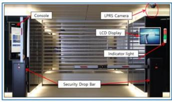
Fig. 8a - Example of Kiosk and Monitoring Devices Outside at the Transfer Cabin
