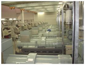
Fig. 22 - Indoor D-UPS Installation
