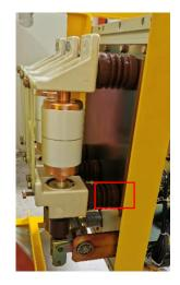
Fig. 28 - VCB Rack Out of the Switchgear Panel
