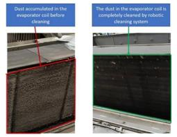
Fig. 4b - Photos showing Before and After Deep Cleaning of ACU Evaporator Coil by Robotic System
