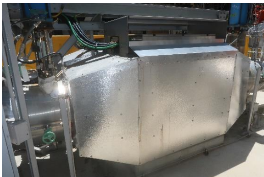
Fig. 7 - Complete Installation of Tapping Flue Gas Electric Heater
