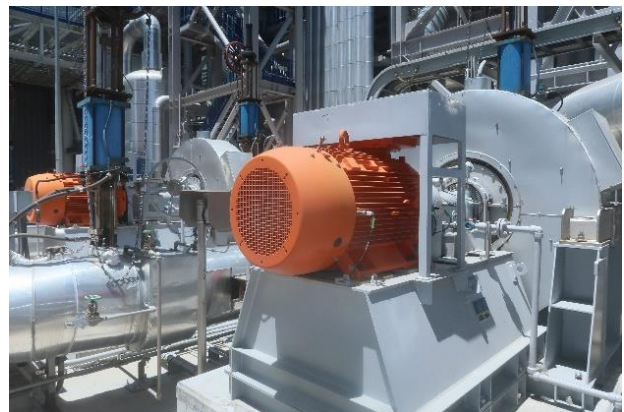
Fig. 6 - Complete Installation of New Tapping Flue Gas Fans
