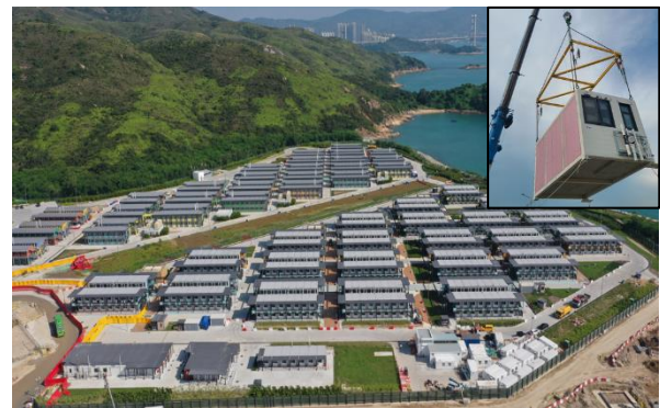
Fig. 22 - MiC Unit at Penny Bay's Quarantine Center, 707 nos. MiC Units Delivered within 87 Days
