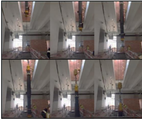
Fig. 28 - Example of Riser Module Hoisting
