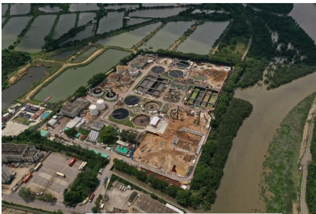
Fig. 3 - Construction of YLEPP
