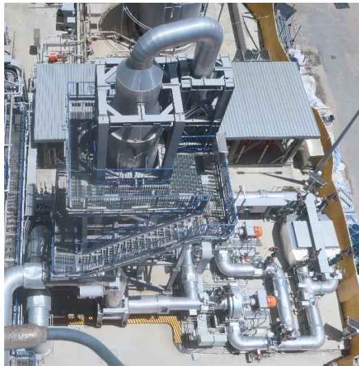
Fig. 4 - Complete Installation of L10 UTAC System
