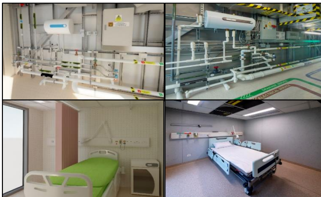
Fig. 25 - MiC Negative Pressure Isolation Ward Fully Designed and Manufactured using BIM
