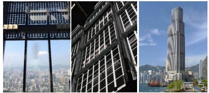
Fig. 5 - BIPV Application at K11 Victoria Dockside, Hong Kong
