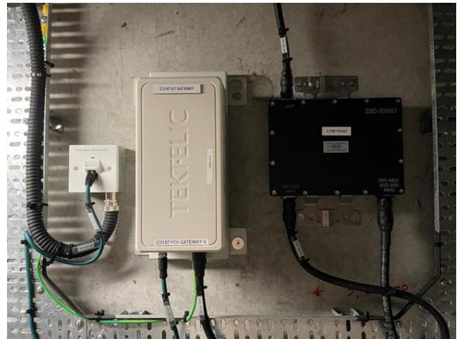
Fig. 3 - Setup of LoRaWAN Infrastructure (Left is IoT Gateway, Right is Point of Interface)
