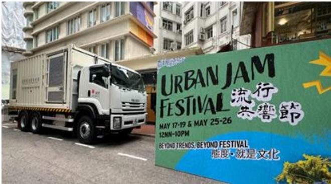
Fig. 12 - Energy Storage Truck (EST)
