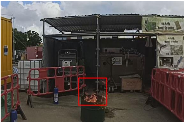
Fig. 7 - Successful Detection of Fire at Worksite During the Trial
