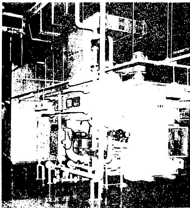
Fig. 3. 66kV, 30000 kVA Gas-only gas insulated transformer (Forced-gas water-cooled)
