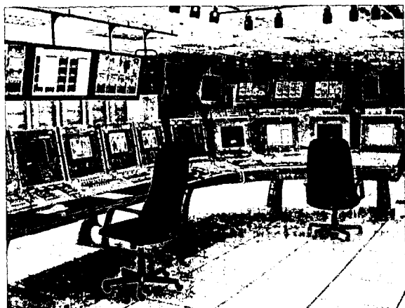
Figure 4 Master Control Room
