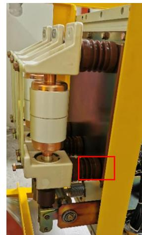
Fig. 28 - VCB Rack Out of the Switchgear Panel
