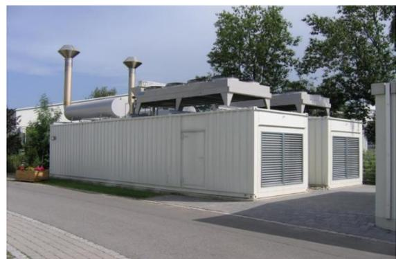
Fig. 24 - Outdoor D-UPS Installation
