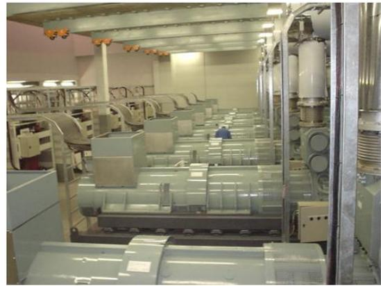
Fig. 22 - Indoor D-UPS Installation
