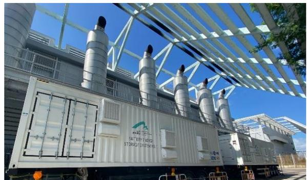
Fig. 7 - Site Photo of BESS in Generator House 1
