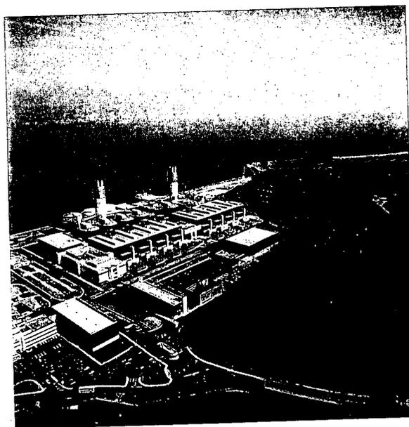
LNG is produced by cooling natural gas to  $-162^{\circ}\text{C}$  ( $-260^{\circ}\text{F}$ ) through a liquefaction process. Prior to cooling and condensing the natural gas into LNG, impurities such as carbon dioxide, water and sulphur are removed. The end result of this process is an odourless, colourless product consisting mostly of methane with small amounts of ethane, propane, butane and pentane.
