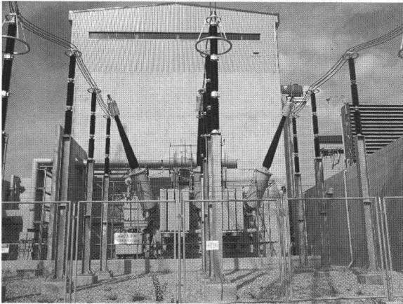
The GT generator is connected to the generator transformer by means of isolated phase busduct (IPB) through GVCB delivering power to the 500kV switchyard. Power from ST generator is delivered to the switchyard in a similar way except without the GVCB. A key single line diagram is shown in Figure 8.
