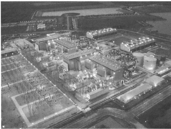
Each block encompass two gas turbines (GT) , two heat recovery steam generators (HRSG), one steam turbine (ST), associated unitized auxiliaries and plant common facilities. Figure 5 shows the Schematic Diagram of a Combined Cycle (CC) Block.
