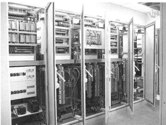
PLCs are utilized for various plant auxiliary processes and linked up with DCS via MODBUS interface for remote control and monitoring in central control room.
